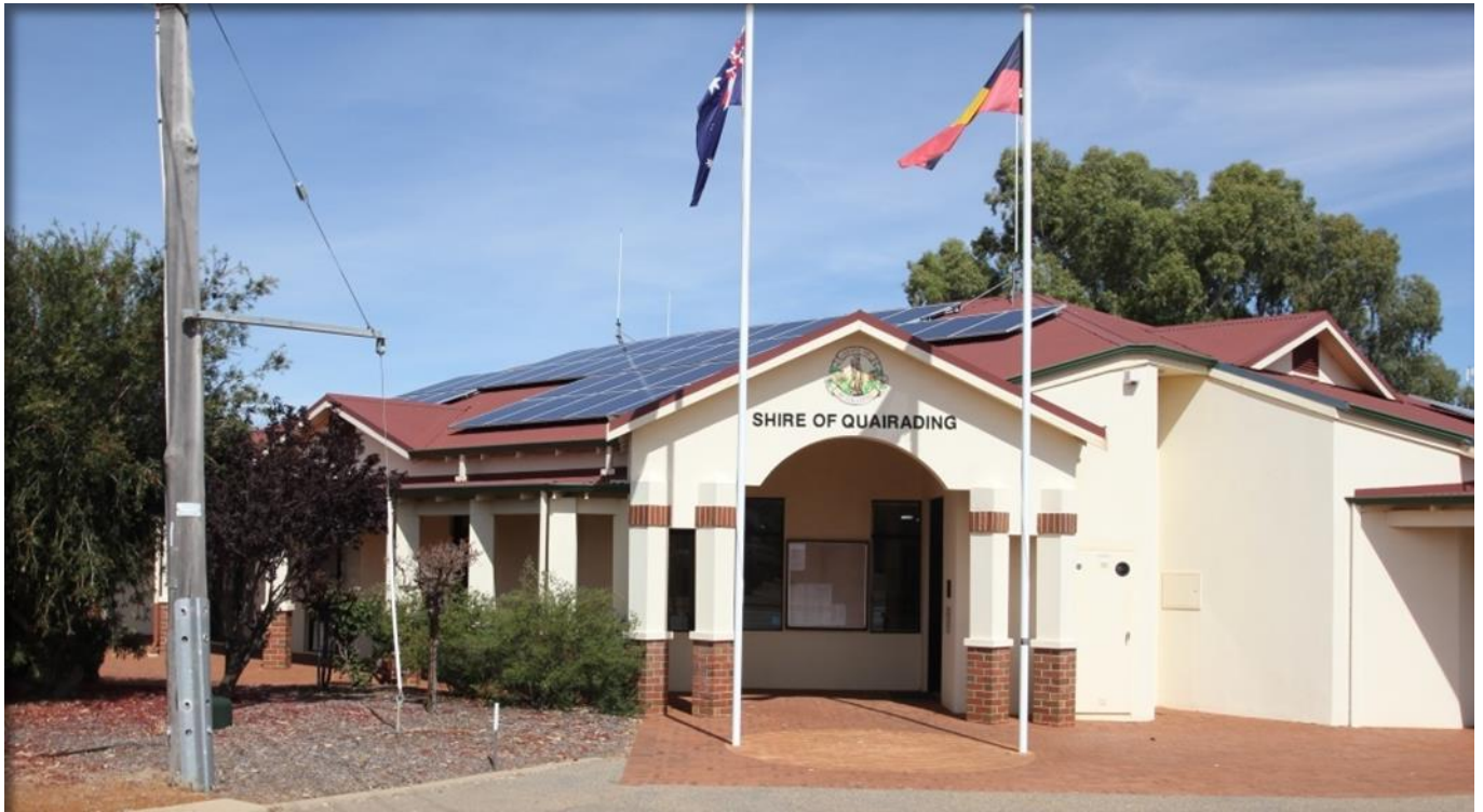
Figure 1 Recent installation at the Shire of Quairading by Solargain
