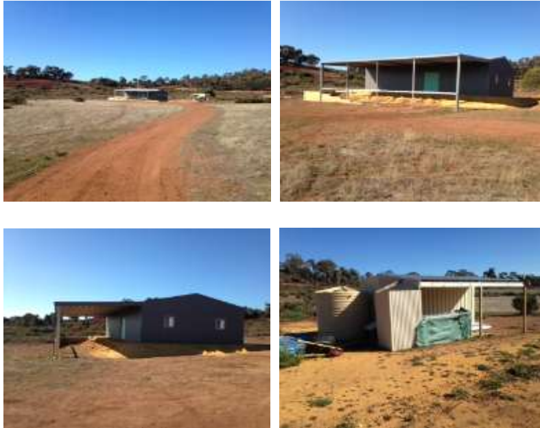
Figure 2 – Photos of partially constructed development
