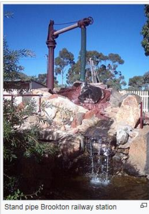
Stand pipe Brookton railway station
